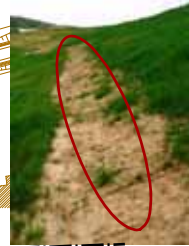
I/ Zone talus STEP
